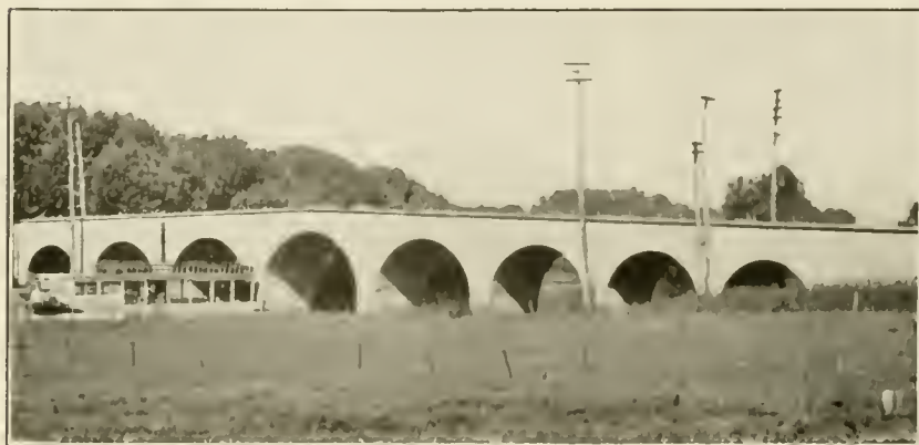
WITMER'S BRIDGE, EAST OF LANCASTER
